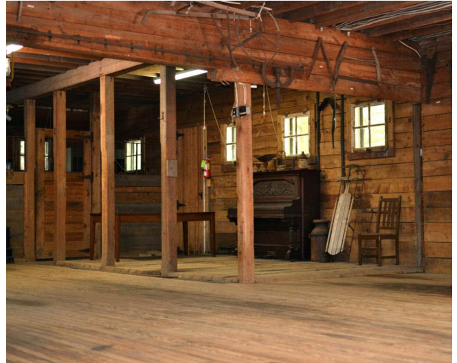
Inside the Carriage House at Lacawac.
