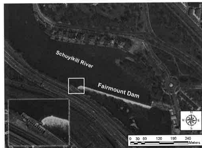
Figure 2. Aerial view of Fairmount Dam and vertical slot fishway (left insert) located on the west bank of the Schuylkill River at river km 13.6, Philadelphia, Pennsylvania.
